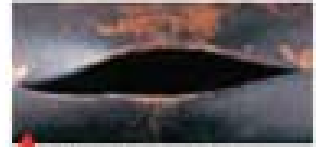
FREEZE RUPTURE Caused by low water flow in the evaporator.
