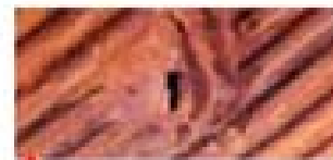
INTERNAL PITTING Caused by an abnormal presence of aggressive elements in water.
