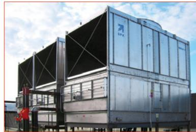
Closed-circuit cooling tower "fluid cooler"
