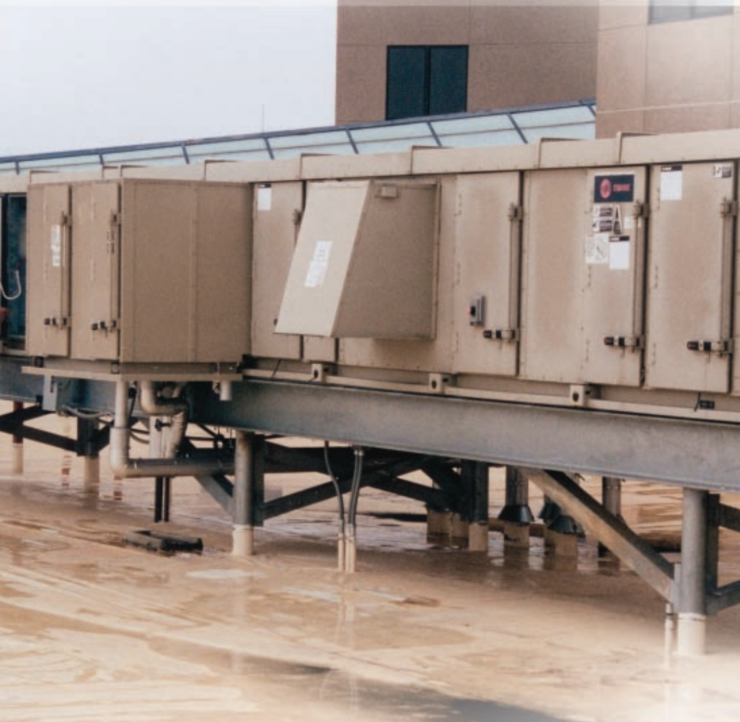
Detached mechanical plant reduces total facility cost and reduces impact of future service or plant expansion activities.
